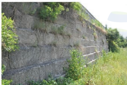
The famous "Eighteen Weirs" embankment near the Pang Village of Yongding River 永定河庞村附近著名的“十八堰”大堤
