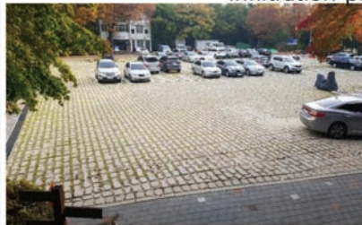
Permeable pavement (Gwangju)
