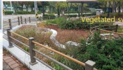
Infiltration planter (Jeonju)
