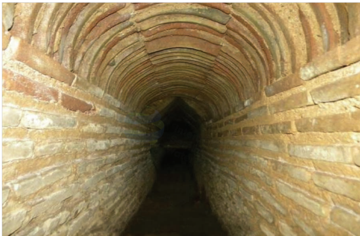
Andrianion aqueduct in Athens
