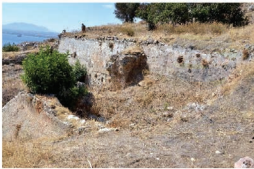
Cistern (of rectangular cross section) in the Palaiokastron in eastern Iraklion used mainly for water supply
