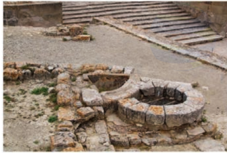
Cistern with sand filter in the "palace" of Phaistos
