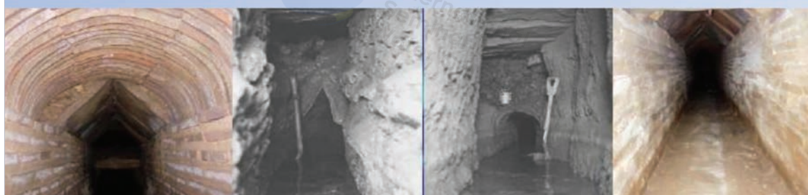
Andrianion aqueduct in Athens
