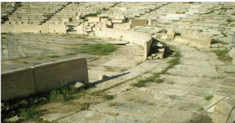
Dionysus theater; details of drainage channel (images by K. Kollyropoulos): (a) view next to orchestra; (b) view of channel exit under stage of theater; (c) view of downwards flow of channel (Kollyropoulos et al., 2015)
