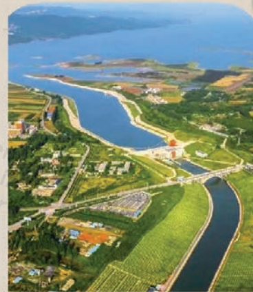
南水北调中线工程“水龙头”——陶岔渠首枢纽 Taocha Canal Headworks – The 'stopcock' of the South-to-North Water Diversion Middle Route Project
