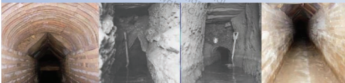
Andrianion aqueduct in Athens
