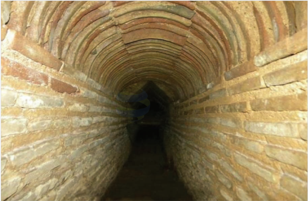
Andrianion aqueduct in Athens
