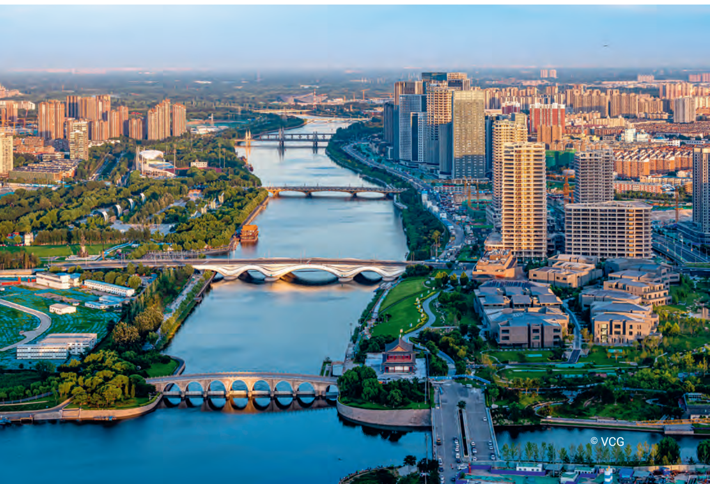
Figure 5-10 The Grand Canal, Tongzhou section in Beijing: The Grand Canal, which had dried up at multiple sections for over a century, has water flowing throughout its course again since 2022
