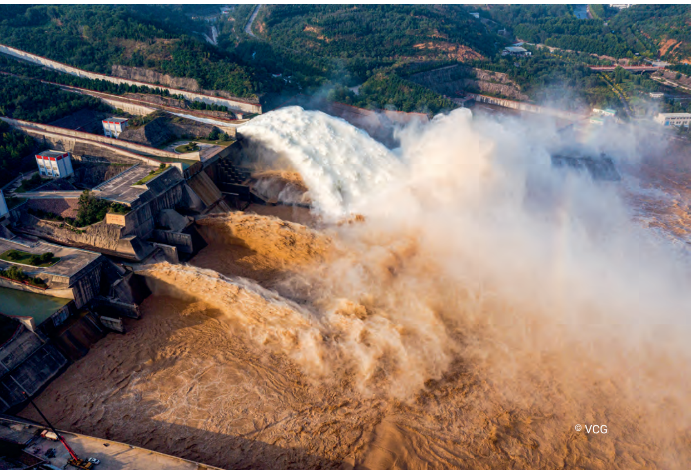
Figure 5-7 Luoyang City, Henan Province: Muddy water gushes out from the sand discharge tunnel during a water and sand regulation operation at the Xiaolangdi Reservoir on the Yellow River
